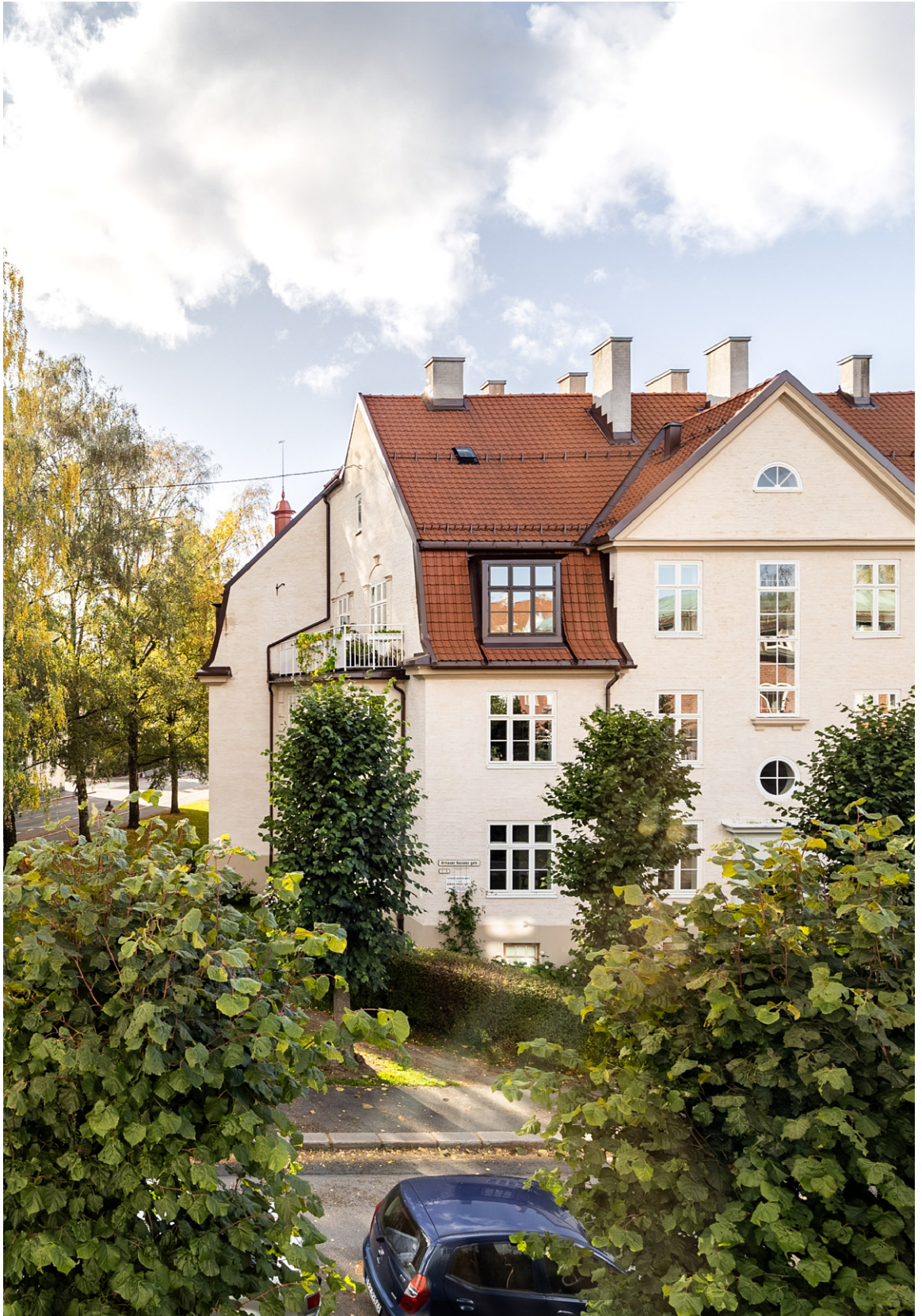
Armauer Hansens gate 1
